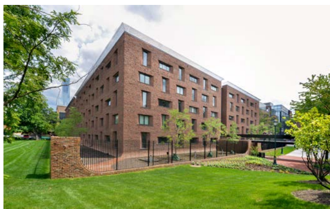
Abb. 235 Fassade [© Aislinn Weidele/Mills + Snoering Architects, LLC.]
